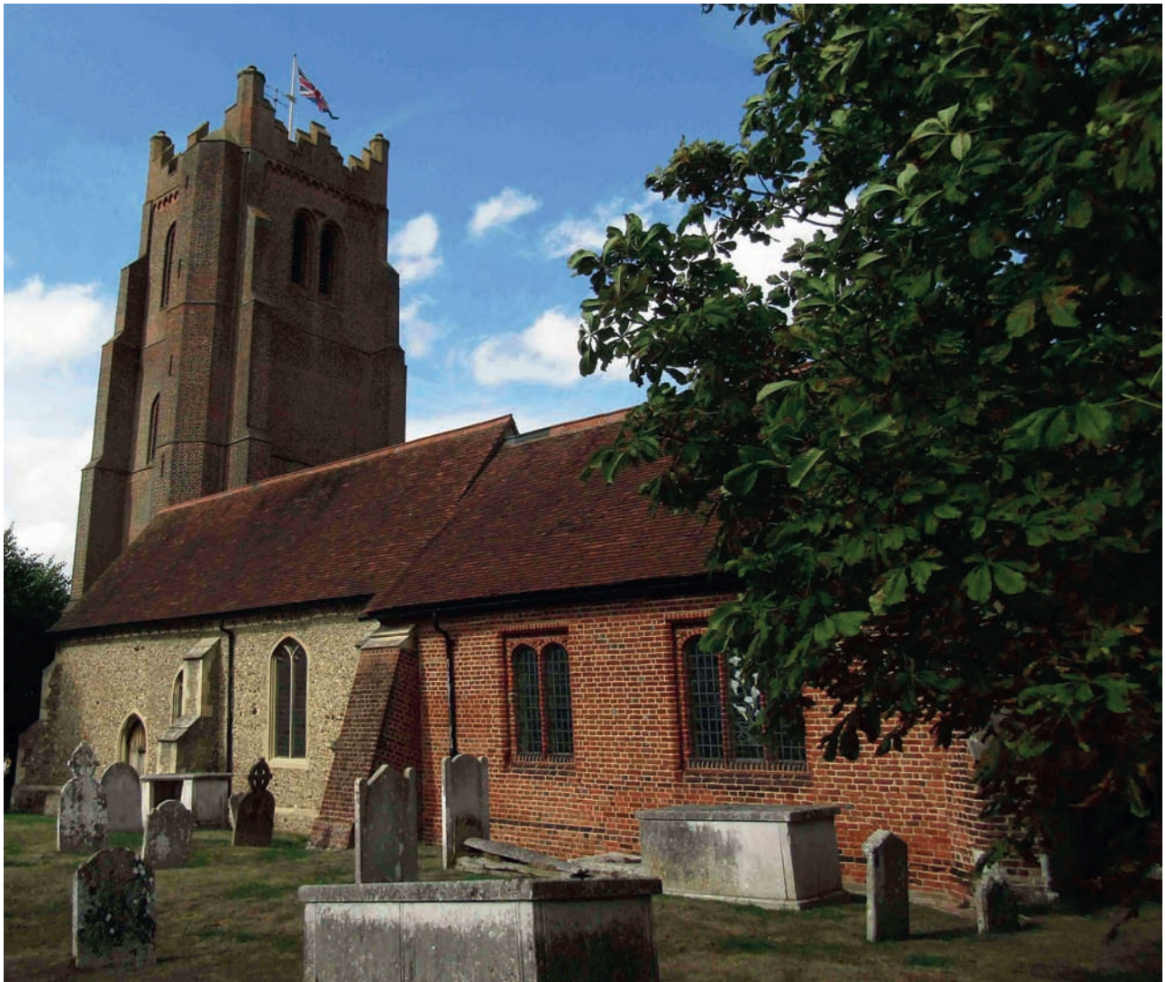
An exterior of Ingatestone parish church with the added almshouse chapel in the same brickwork as the contemporaneous cottages nearby.
