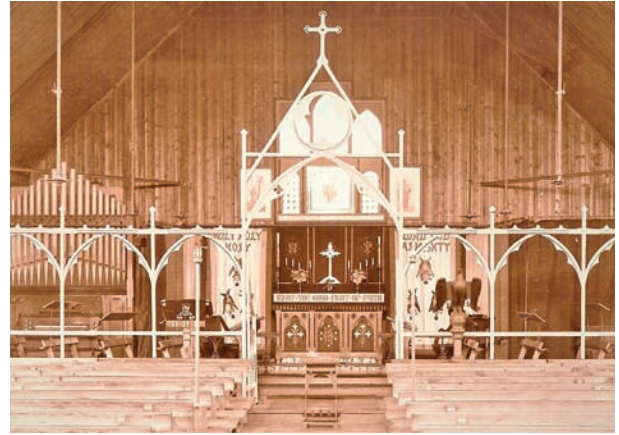
All Saints Church interior view
