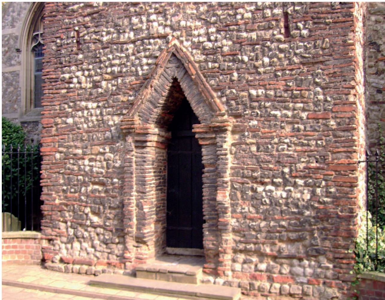
Roman building materials were still readily to hand when the doorway to Holy Trinity church was constructed in the centre of Colchester, possibly around 1050 AD
