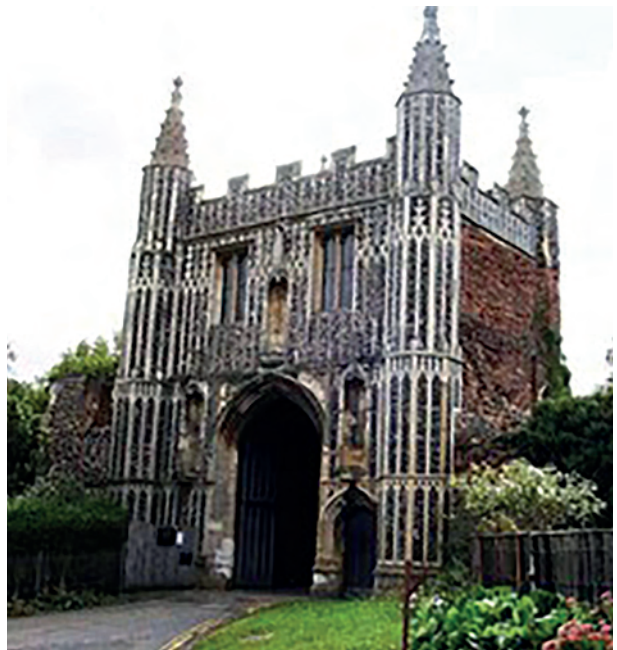
The surviving gatehouse of St John's Abbey
