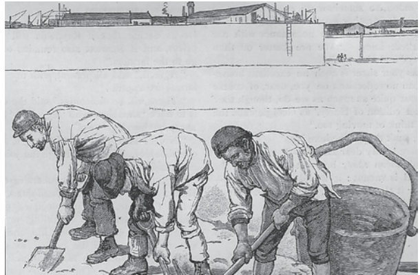
Main dock construction at Tilbury. Cassells Family Magazine 1886 p.221. Author's collection.
