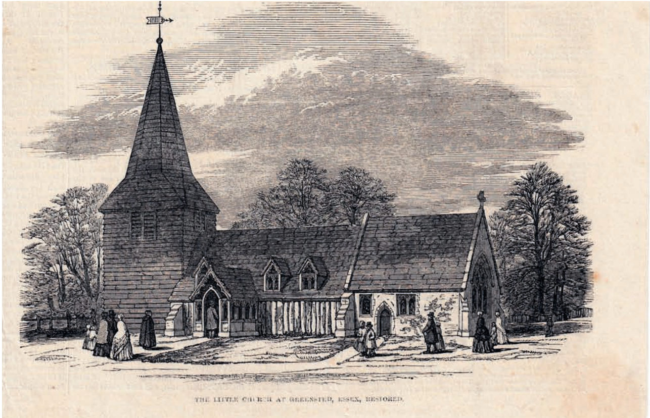
Greensted church from the south after restoration. Note re-arrangement of the nave buttresses, additional and rebuilt dormer windows, and reconstructed porch (Illustrated London News of 3 March 1849)
