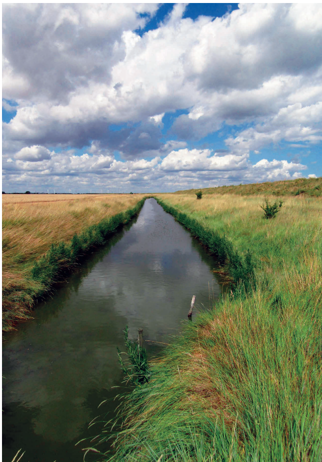
Borrow Dyke and Sea Wall today
